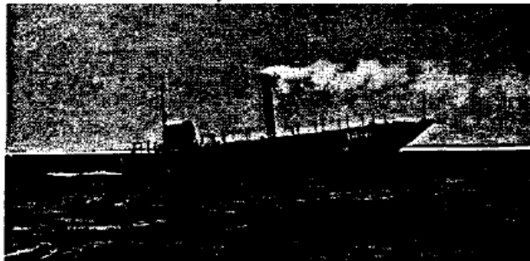
FIG. 2. Landing craft, Model LCM-8, emitting oil-fog smoke.
