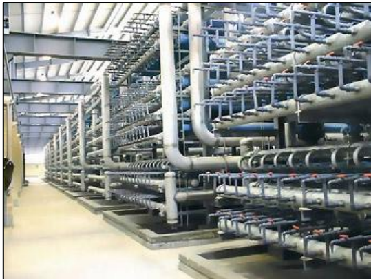
Reverse-osmosis plant, up to 1000psi operating pressures, courtesy water-technology.net
