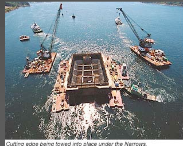
Cutting edge being towed into place under the Narrows.
