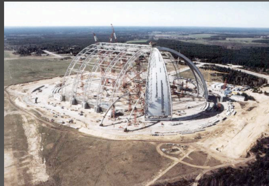
Blimp hanger built to demonstrate construction method for new confining shelter
