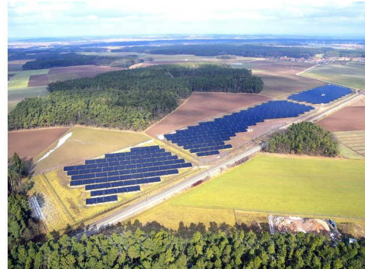
3.1 MWp of CIS modules near Bonnhof, Germany (Solar Frontier)
