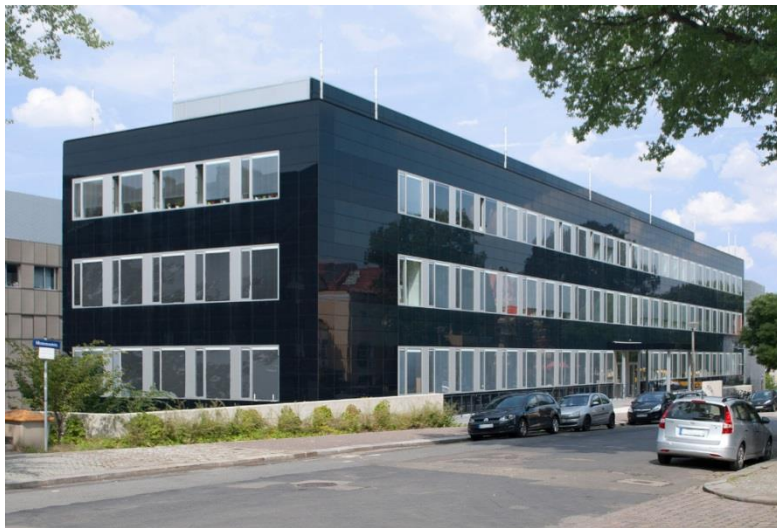
Building integrated CIGS with 500 m 2 (Manz AG)
