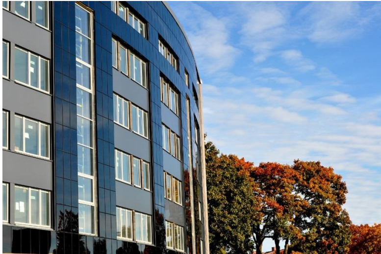
Building integrated CIGS modules in Sweden (Solibro)
